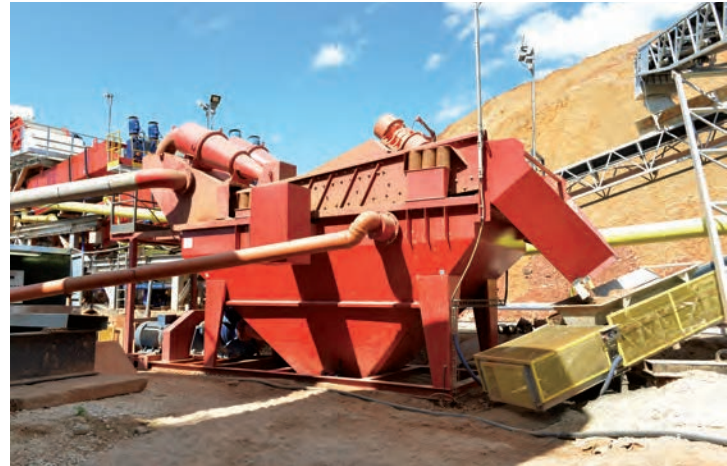
Aggregates and sand with bentonite recovering
